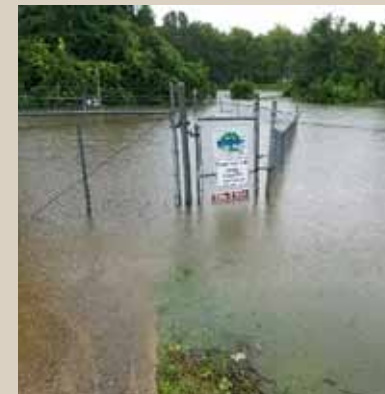
Oyster Creek Flood Level off Mason Near Elevated Storage Tank
