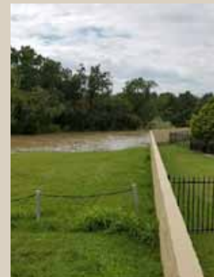
Jones Creek @ the South Side of Pecan Lakes Flood Wall
