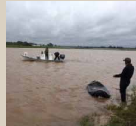
Dive Team Installing 60" Plug at Plantation 4/5
