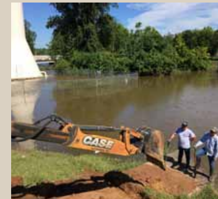
EDP Performing North Pump Station Box Culvert Repair
